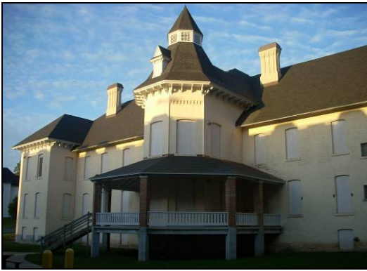
Completed Roof Renovation
